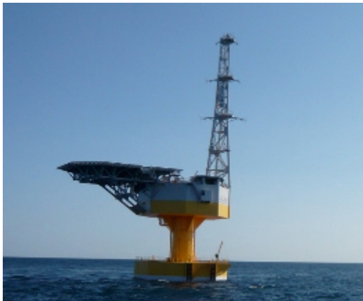
The 66kV floating substation at Fukushima Kizuna; Image via Marubeni
