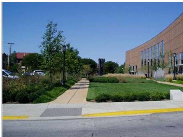
A bioswale of native plants at Purdue University, show here at the right of the parking lot, collects storm water run-off and allows it to filter into the soil. (Don Staley/Purdue University)
