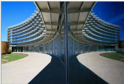
The Applied Research and Development facility at NAU has an exposed frame of concrete, which stores thermal energy and provides 50 percent of the building's heating requirements. (Northern Arizona University)
