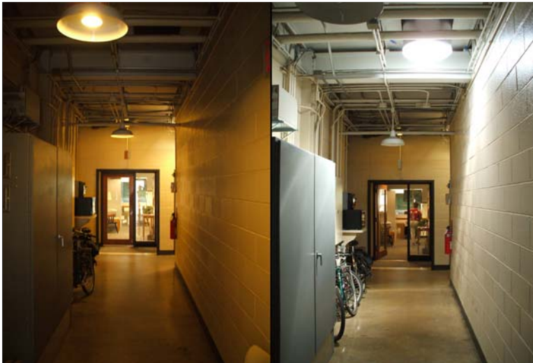
These before-and-after shots show the dramatic difference that reflected sunlight makes to a dark hallway. (Princeton University, Facilities Organization, Arthur Murphy)
