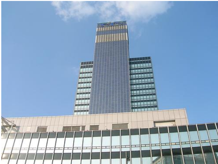
CIS Tower in London, UK with BIPV built into the smart façade via Flickr Gene Hunt
