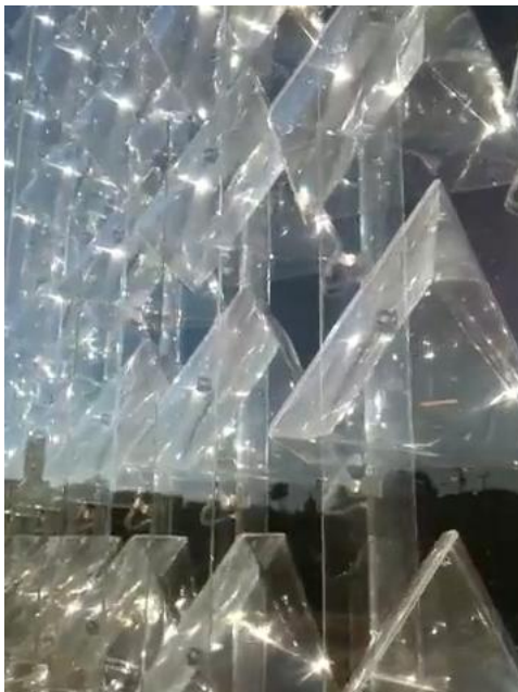
HeliOptix Integrated Concentrating Solar Façade System at SyracuseCoE
